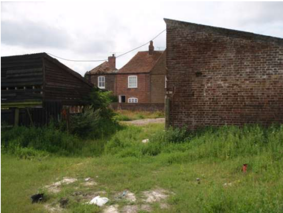
Plate 8. View across the farmyard south to the Farmhouse (looking south)
