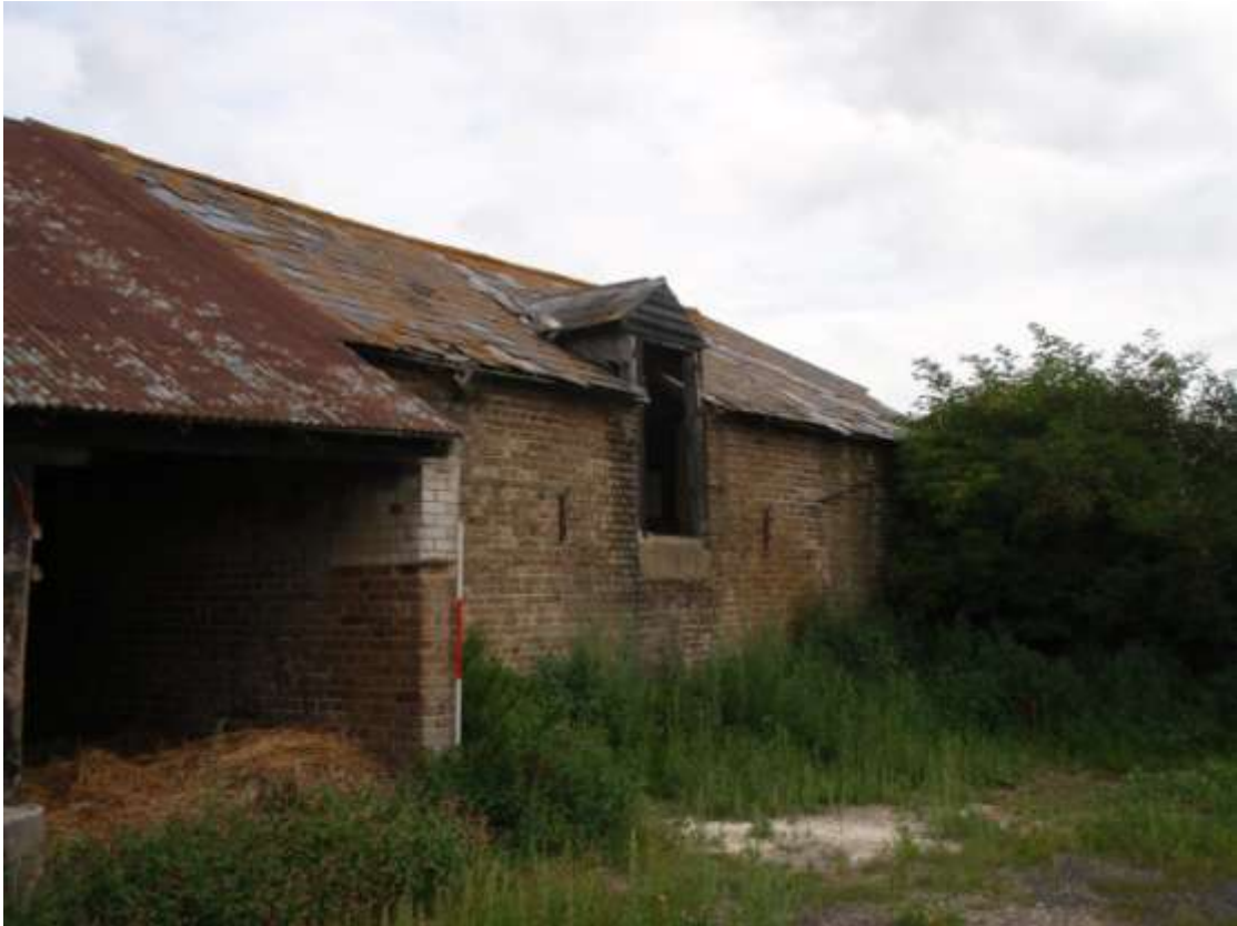
Plate 10. View of the Granary Building (looking NE)
