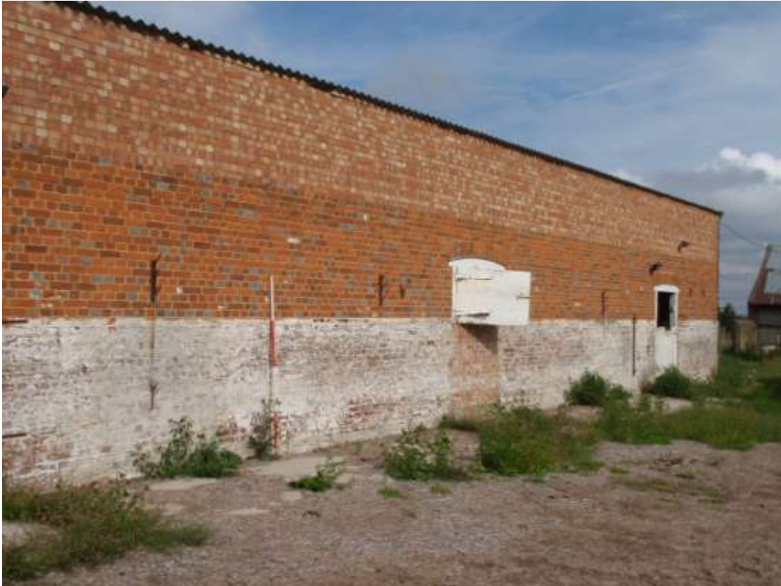
Plate 20. View of Livestock Building (looking NW)
