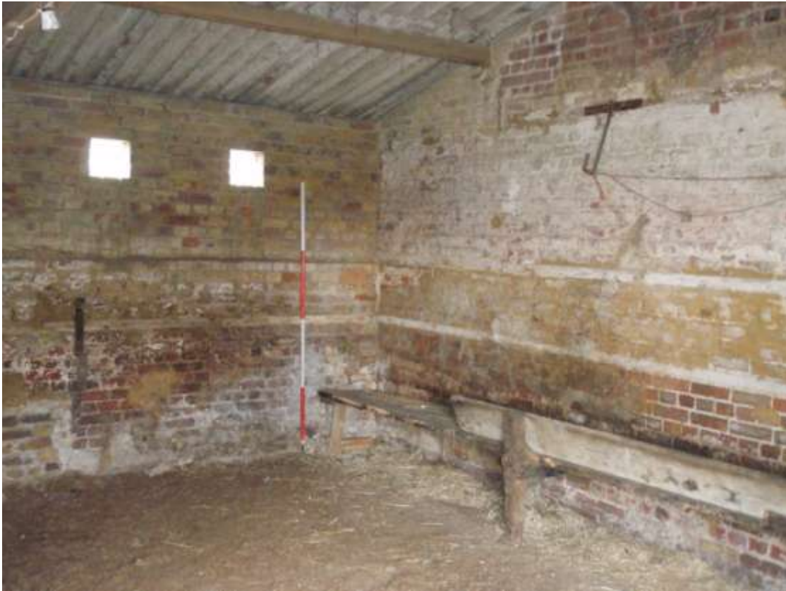
Plate 21. View of inside Livestock Building (looking NW)
