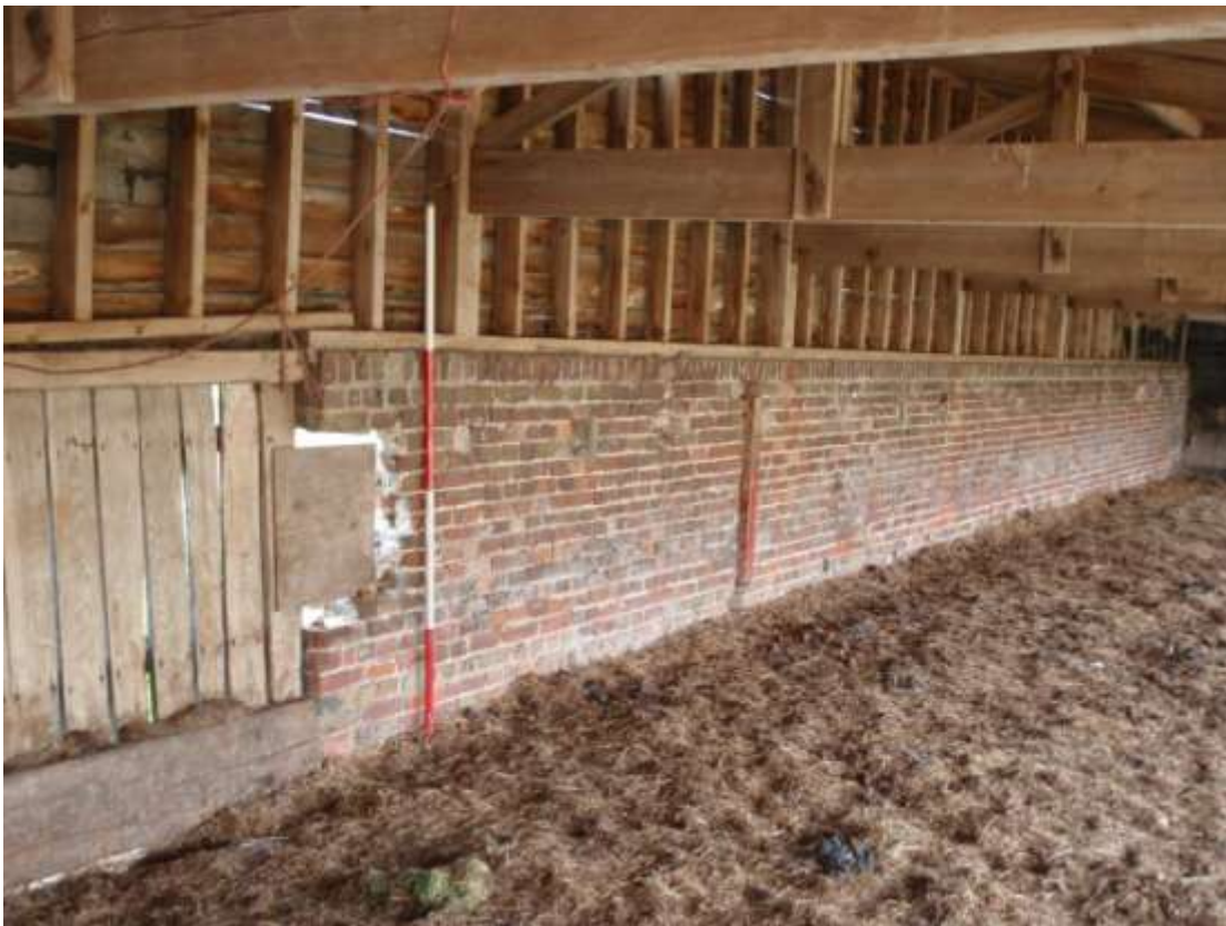
Plate 26. View of the interior of Cart Shed Building (looking NE)
