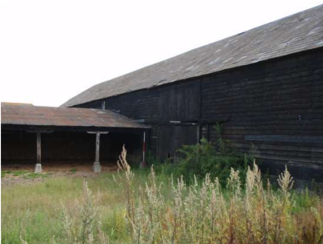
Plate 28. View of Cart Shed Building (looking NE)
