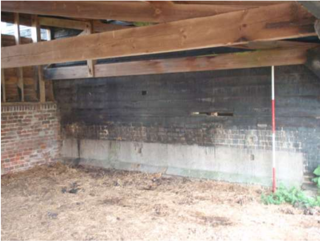
Plate 27. View of the interior Cart Shed Building (looking NE)
