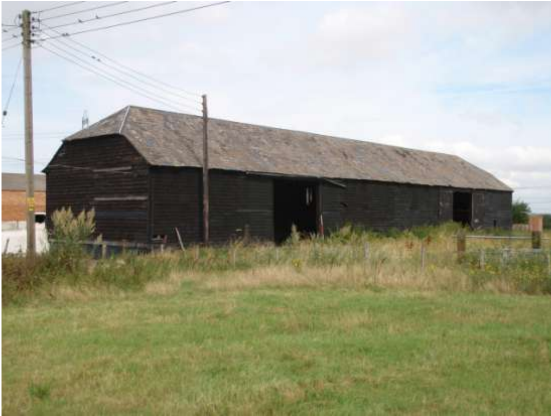
Plate 15. View of the east facade south end of the Barn (looking NW)
