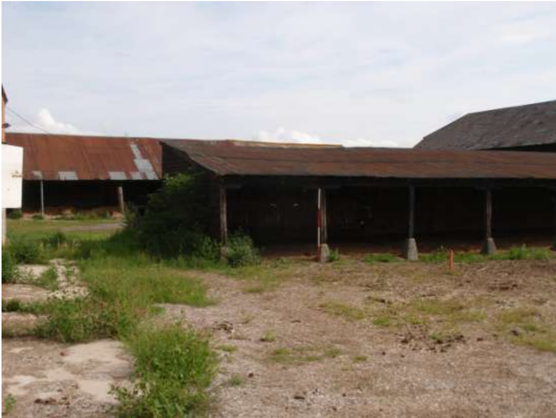
Plate 25. View of Cart Shed Building (looking NE)
