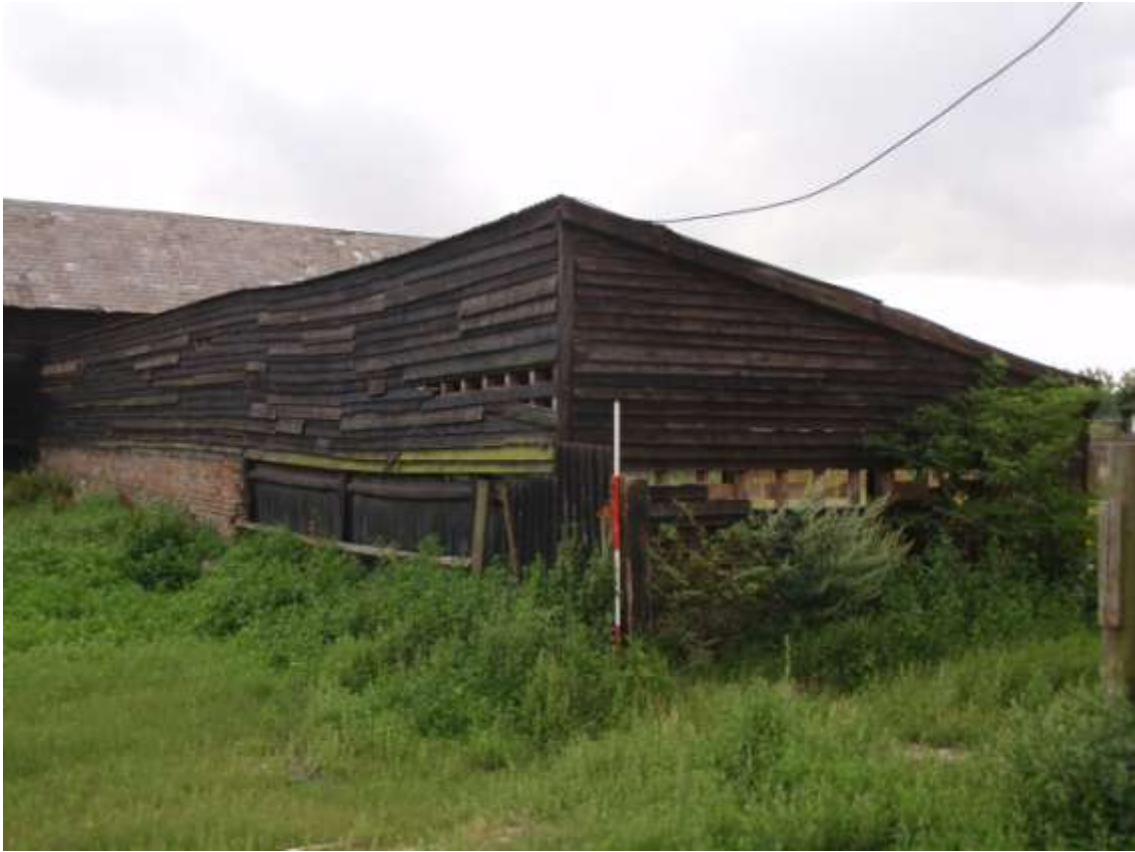
Plate 29. View of Cart Shed Building (looking SE)
