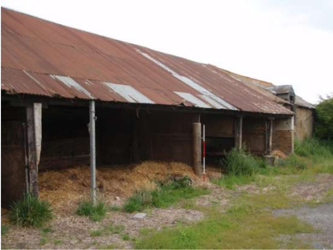
Plate 9. View of the Granary Building and adjacent Livestock Pens and Cart Sheds (looking NE)
