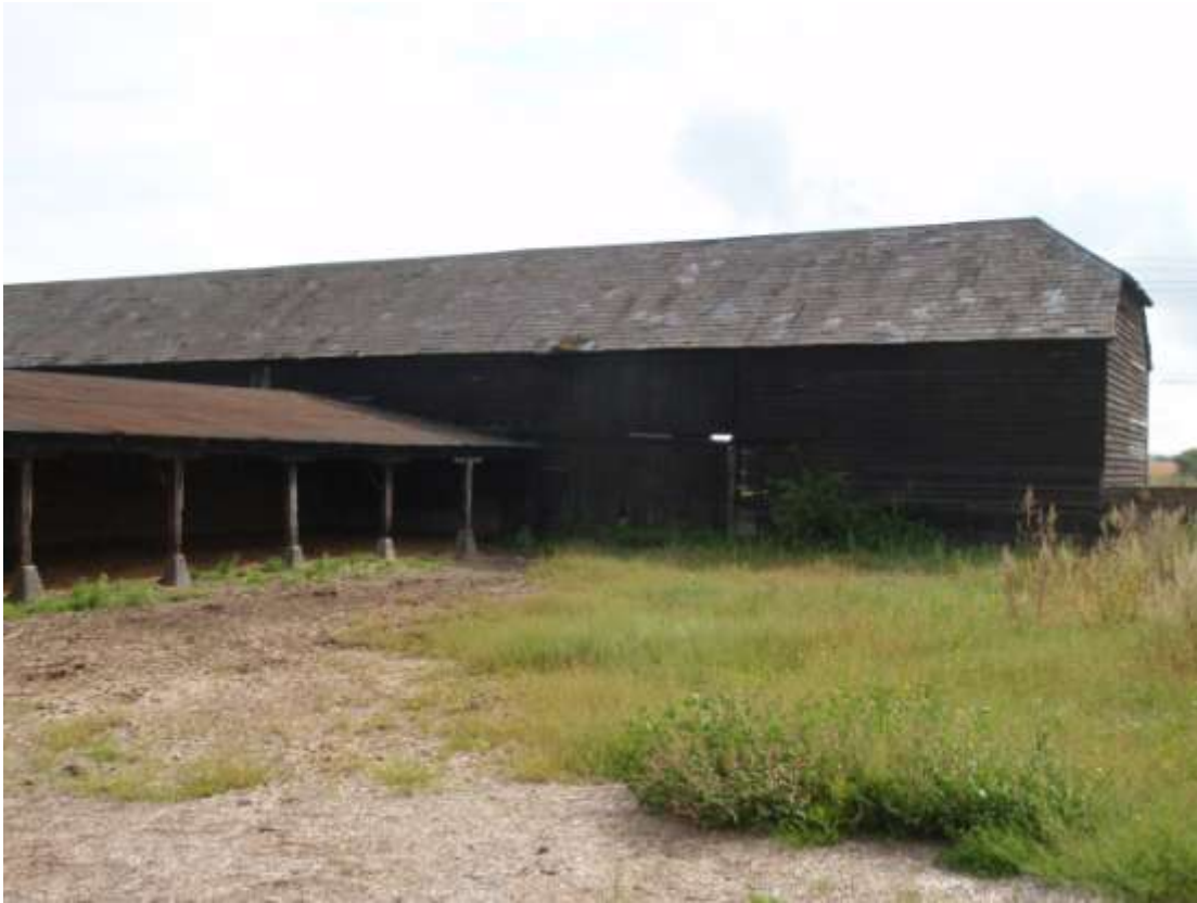
Plate 23. View of Cart Shed Building (looking NE)
