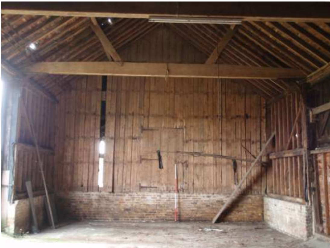
Plate 16. Inside view of Barn (looking south)
