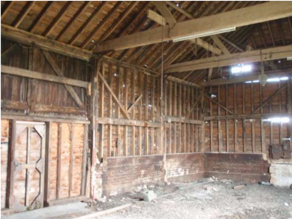
Plate 18. Inside view of Barn (looking NW)
