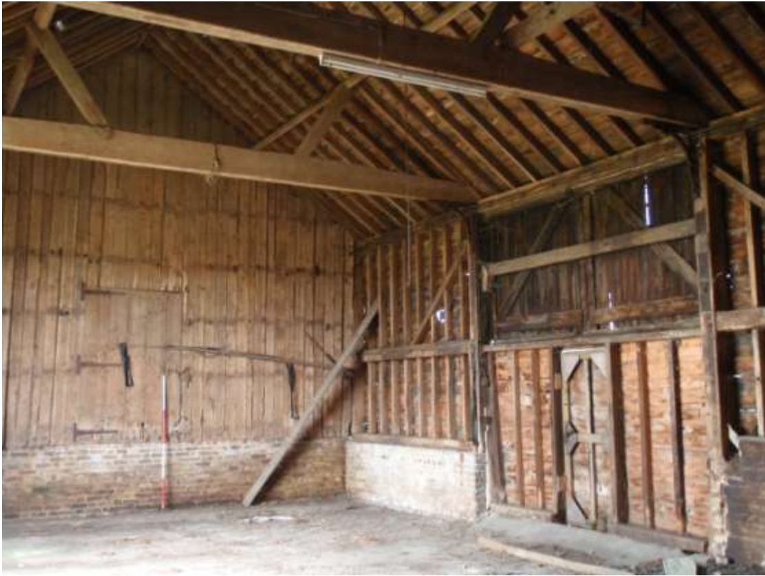
Plate 17. Inside view of Barn (looking SW)
